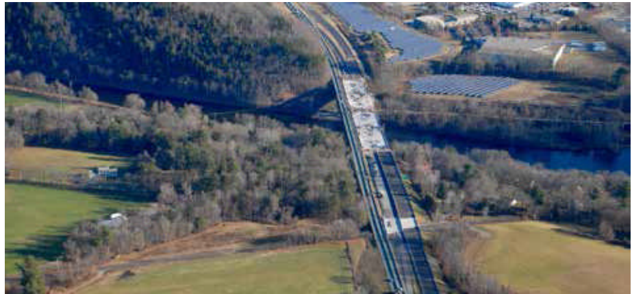
BRATTLEBORO. Two aging steel bridges are being replaced with a single concrete span on I-91.
