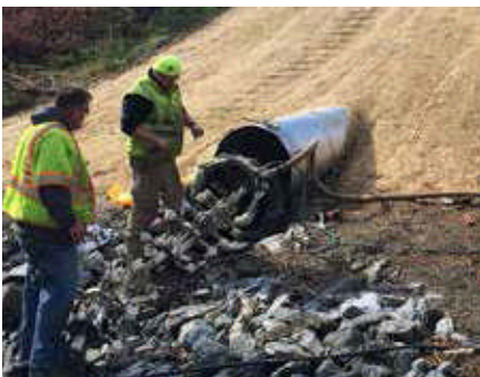
VTrans employees install a culvert liner. Liners are cost effective solutions for prolonging the life of culverts.
