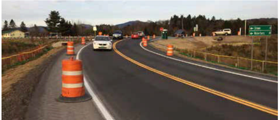
MORRISTOWN. Fresh pavement before the installation of a new signal on VT 100 in Morristown.
