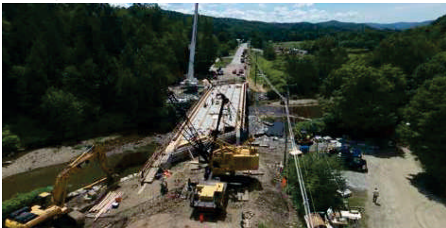
WAITSFIELD. Construction of a replacement bridge over the Mad River along VT100 in Waitsfield. The new bridge is being constructed using Accelerated Bridge Construction methods to minimize the length of the bridge closure.
