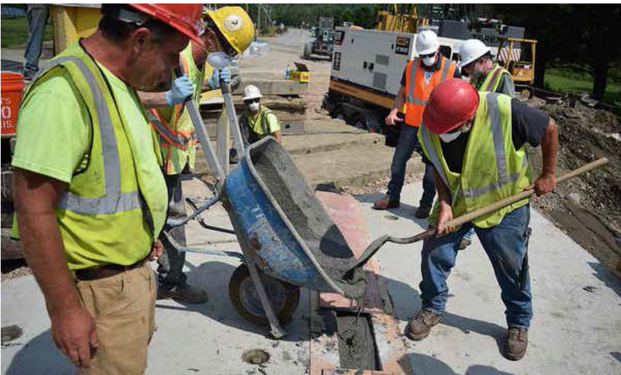
The VT100 bridge project in Waitsfield is the first use of Ultra-High Performance Concrete in Vermont. UHPC provides added resilience over traditional concrete.
