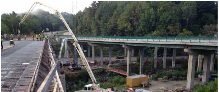
WATERBURY. Construction of I-89, Exit 10 north bound off-ramp bridge.
